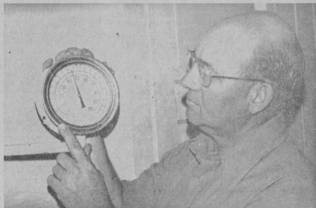
WATER PRESSURE at the city hall was around 47 pounds when this picture was snapped Tuesday afternoon. City Mgr. Reginald Bublitz said he had asked several large water users to stop the sprinkling of lawns and the pressure jumped four pounds in a short time.—Tawas Herald Photo.
