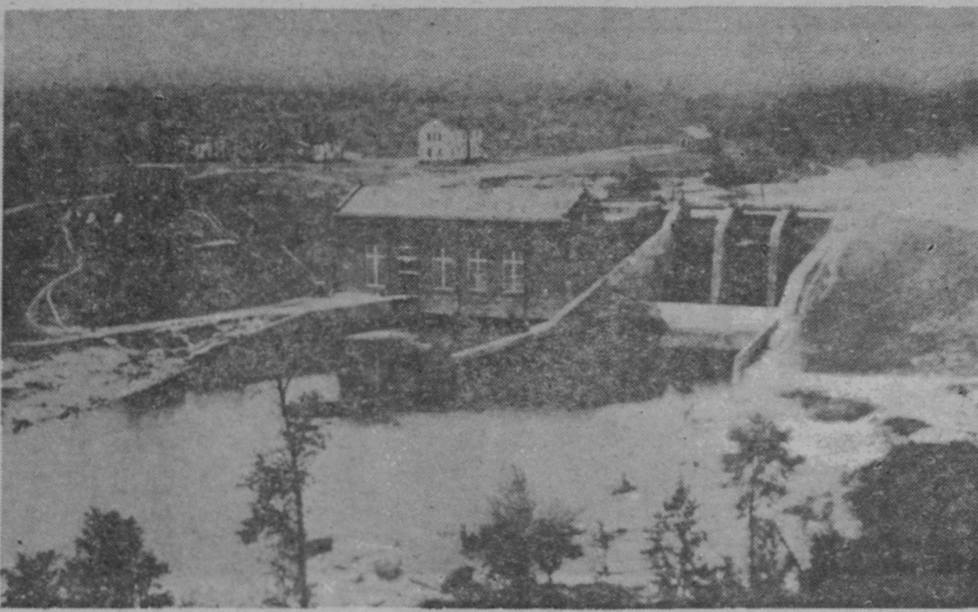
COOKE DAM went into service in 1912 as the first hydroelectric generating plant on the AuSable River and opened a new era in the history of Eastern Michigan.
