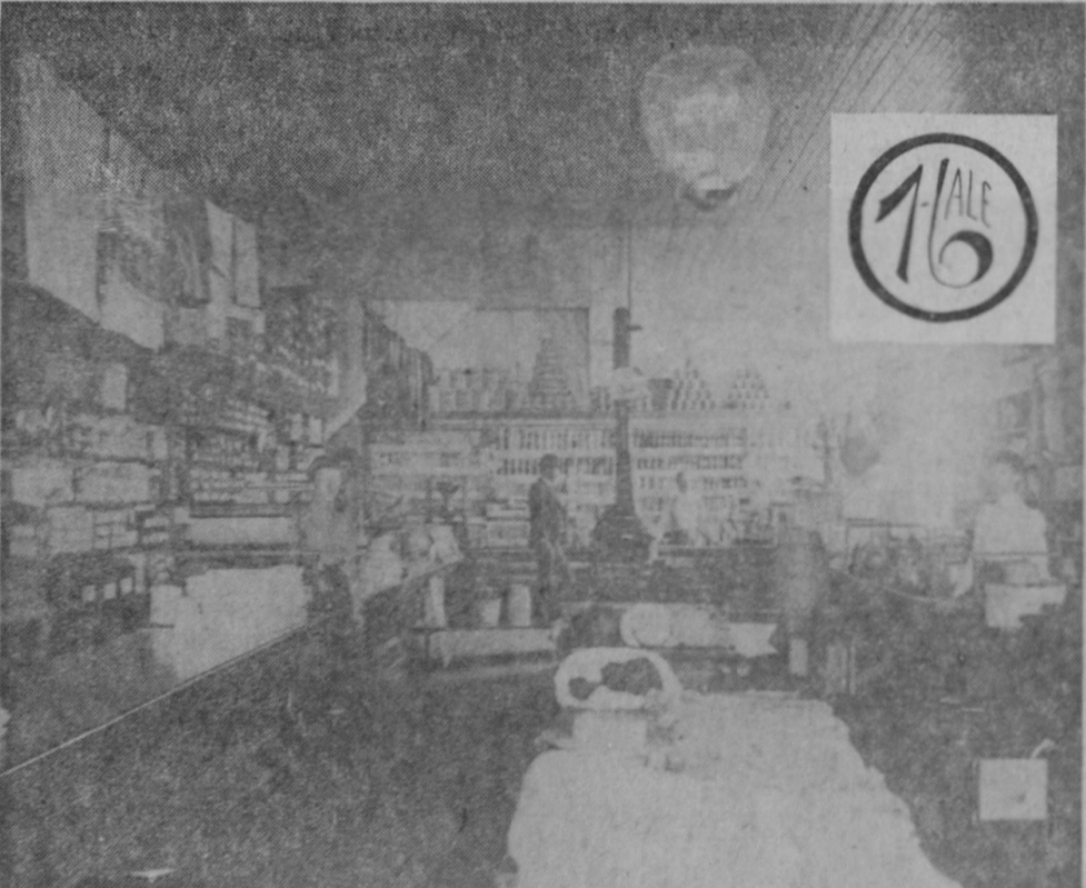
HERE'S A PICTURE OF THE INTERIOR OF YAWGER'S STORE PRIOR TO 1900.
