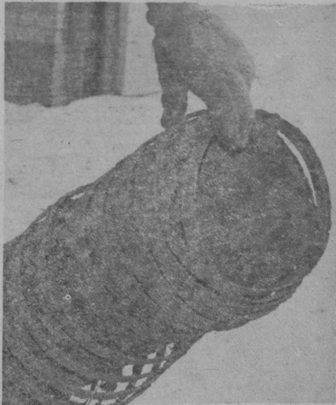
A SECTION of the iron banded wooden pipe which once conveyed salt brine from East Tawas to AuSable-Oscoda is pictured here. —Tawas Herald Photo.
