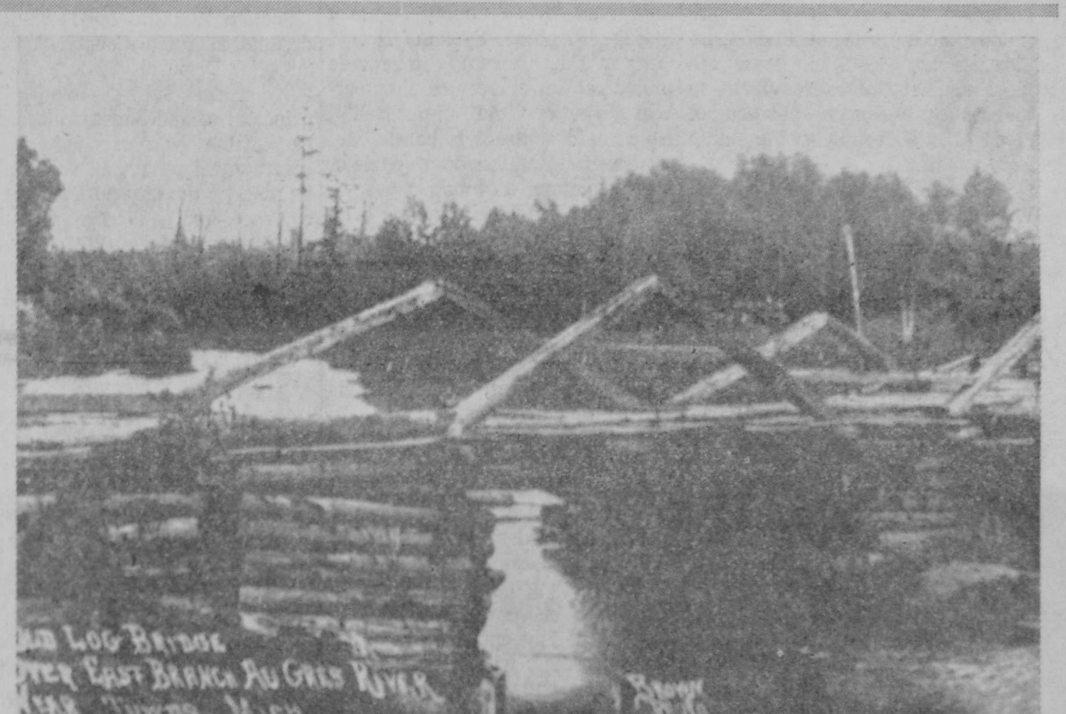
BRIDGING STREAMS has always been a major undertaking in road construction. The primitive log bridge in the above picture spanned the East Branch of the AuGres River for many years before being replaced by this concrete arch in 1909. The latter bridge was constructed by Grant
