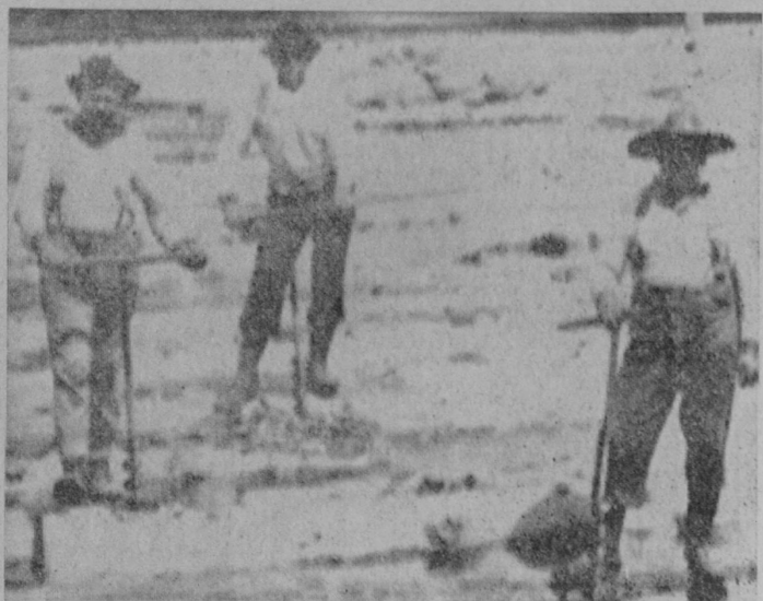
LOG RAFTS were formed in Canada by chaining logs end-to-end to make a circular enclosure. This "bracelet" surrounded a floating mass of logs which was then towed by one or more tug boats. The men in the photo are drilling holes in the logs to admit large chains in the log rafting procedure.
