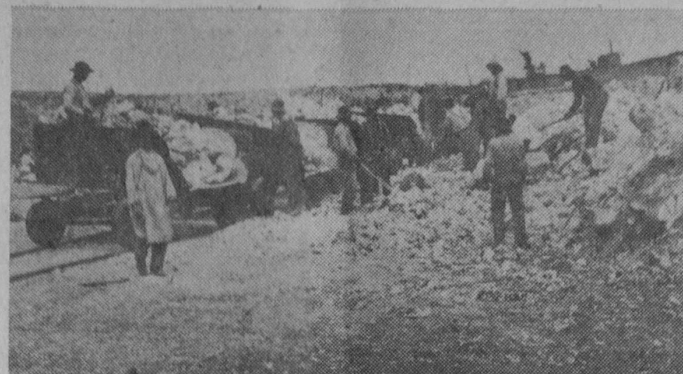
Alabaster gypsum quarry around 1905.
