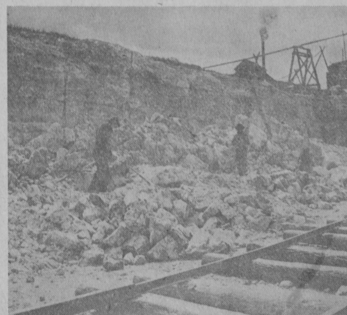
MANY CHANGES have taken place in strip mining at Alabaster since this picture was taken. Hand forks first moved gypsum rock, followed by steam shovels, which were later replaced by electrically powered monsters. A conveyor system now transports both rock and overburden.
