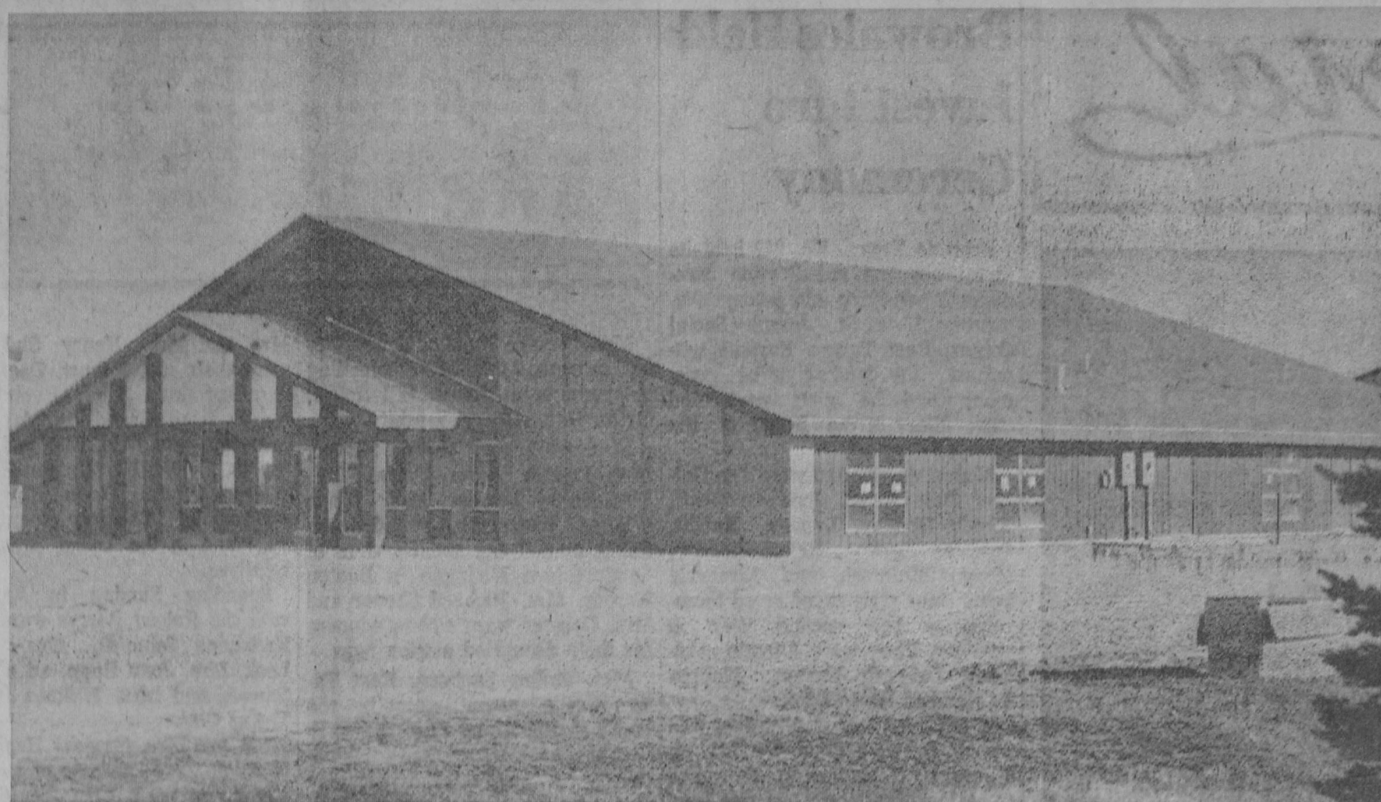
NEARING COMPLETION at Hale is the new home of Bernard Lumber Company. The firm had planned to open in its new quarters by January 1, but construction is running ahead of schedule. Shown above is the new 96 by 100-foot sales and display showroom, constructed of brick and steel. Two 100 by 100-foot storage buildings are under construction and six 36 by 80 foot storage sheds
