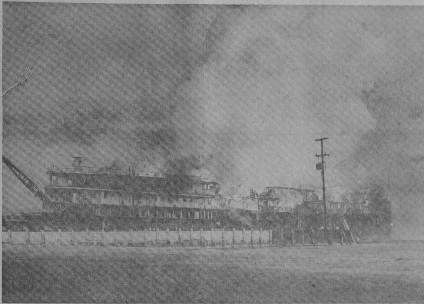
THE SS WESTERN STATES provided the Tawas with one of the most spectacular fires in area history when it burned on March 21, 1959. Said to have been caused by a torch used in scrapping operations, the ship was turned into an inferno and was demolished in a matter of minutes. Several minor fires had broken out during scrapping operations.—Tawas Herald Photo.
