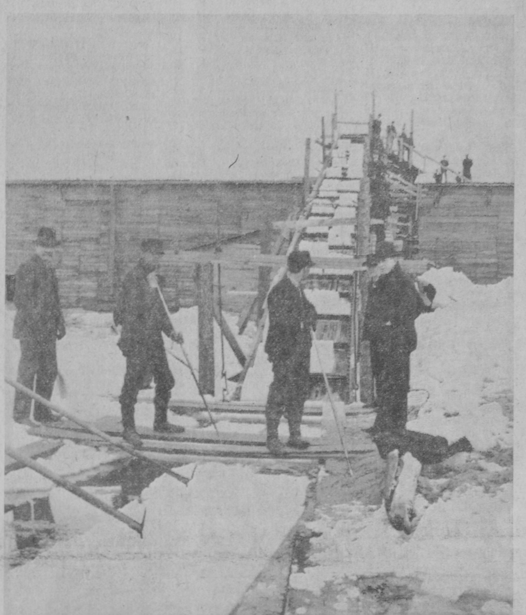
HARVESTING ICE was big business on Tawas Bay in the early 1900s. This picture by A. G. Emery shows men with pike poles pushing cakes of ice onto a conveyor system which transported the blocks of frozen water to the storage building in the background. A Cleveland, Ohio, firm constructed two large ice houses on the shore of Tawas Bay in 1909. Train loads of ice were shipped to market each winter and nearly 300 men were employed in the cutting operation.
