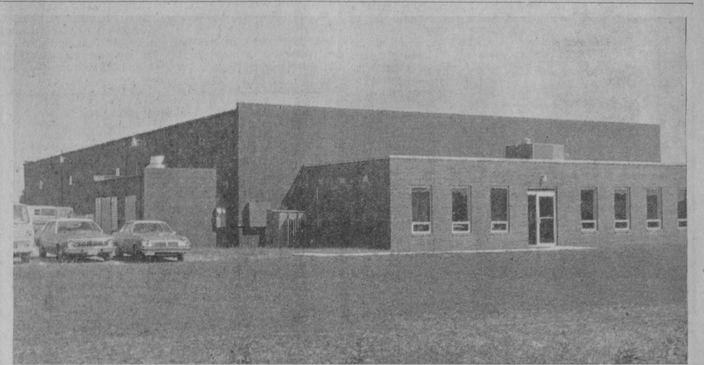
THE NEW Whittemore plant of Valeron Corporation is pictured above. Work started on the structure last fall and was completed a
