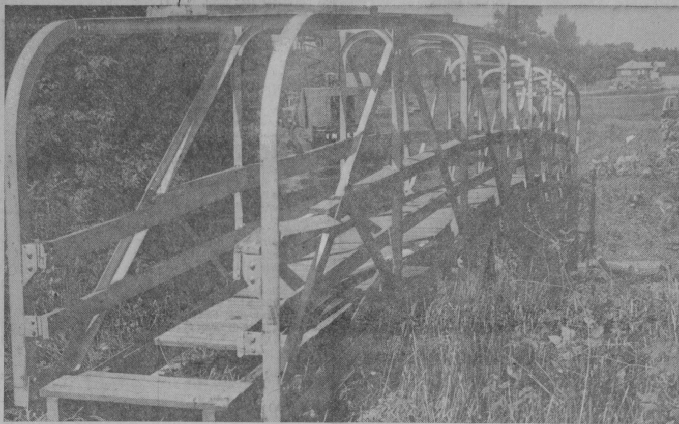
AN OLD IRON and wooden walkway which was salvaged when the Mathews Street bridge was replaced a number of years ago has been installed as a footbridge over Dead Creek on Ninth Avenue. This picture was snapped Wednesday afternoon after department of public works and CETA employees moved the bridge from its storage spot at the city garage about two blocks away to its new location. Concrete footings are to be poured and the bridge is to be moved to its permanent location. A number of wooden beams in the structure are to be replaced. When completed, the bridge will permit youngsters to cross directly to grounds of Tawas City Elementary Unit, saving several blocks of walking.—Tawas Herald Photo.
