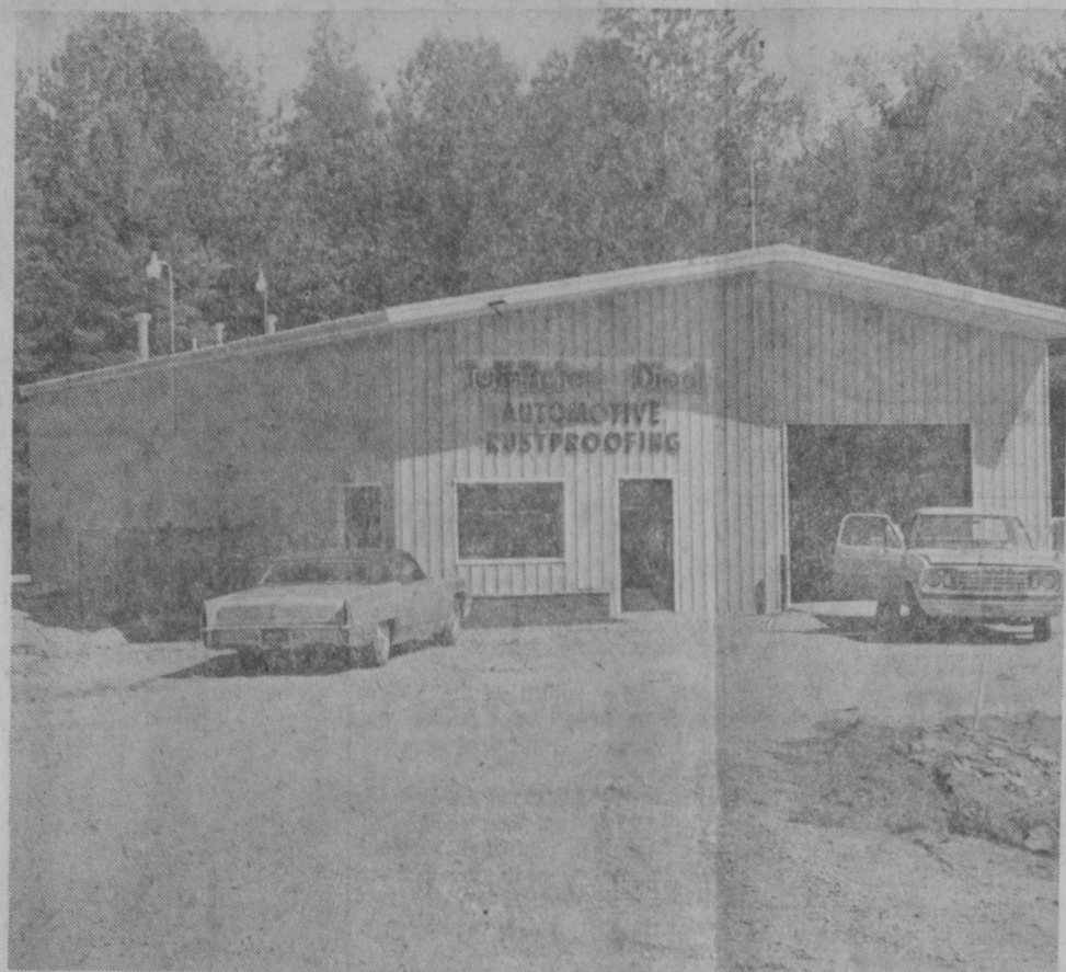
GRAND OPENING is being held for the new Tuff-Kote Dinol automotive rustproofing business owned by Hayes Enterprises on US-23 south of Tawas City. Construction was completed recently on the new building pictured above.—Tawas Herald Photo.
