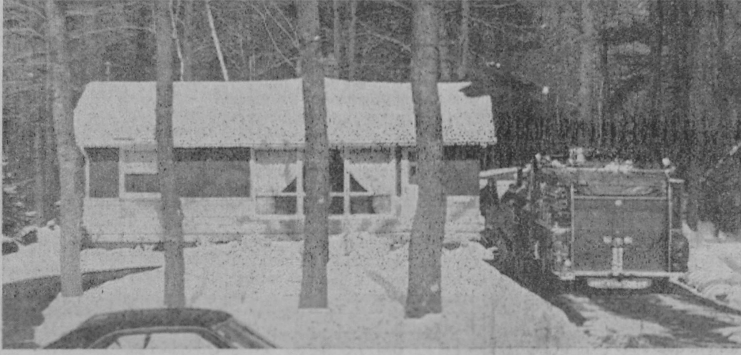
EAST TAWAS firemen answered a call Sunday morning at the residence of Granville Beatty on East Bay Street. The home owner was thawing frozen water pipes with a blow torch and minor damage was caused by the fire. It is expected that such fires will increase in the days ahead due to freezing weather and extreme caution is urged in thawing pipes.—Tawas Herald Photo.
