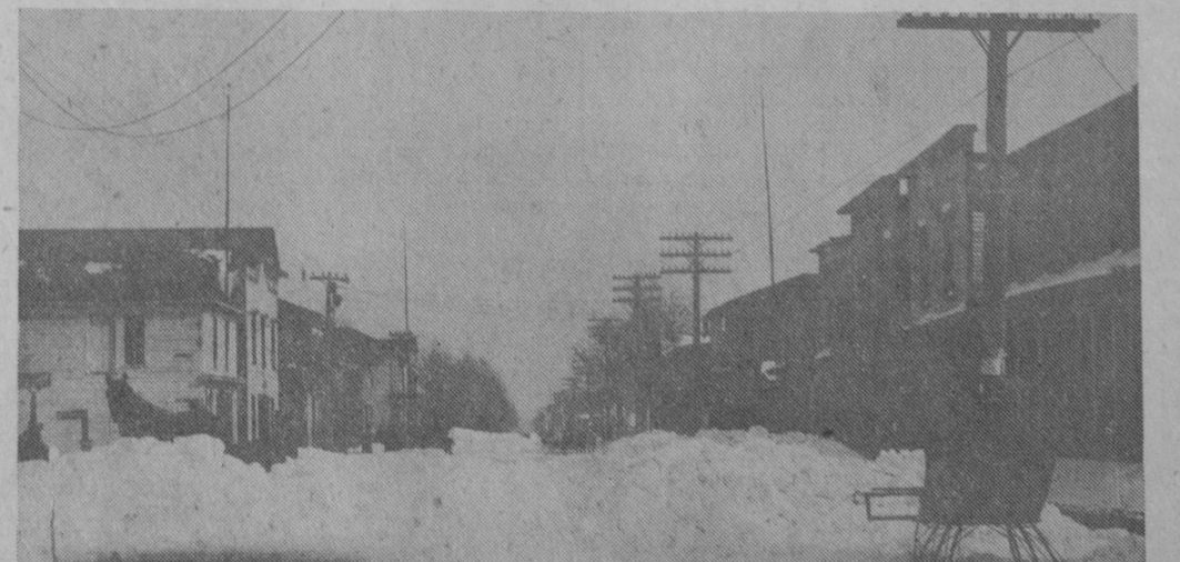
TAWAS CITY'S Lake Street was plugged with snow in this picture snapped in 1908. A lone cutter stands at the southeast intersection with Mathews Street and the owner has taken his
