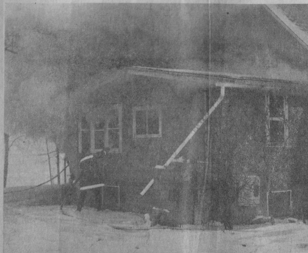
FIRE late Thursday afternoon destroyed the residence of William Neumann on Bay Drive, Alabaster Township. Neumann was visiting at Detroit and flames were spotted by a neighbor. Tawas City Fire Department, assisted by East Tawas firemen, battled the blaze in below zero temperature for about three hours.—Tawas Herald Photo.
