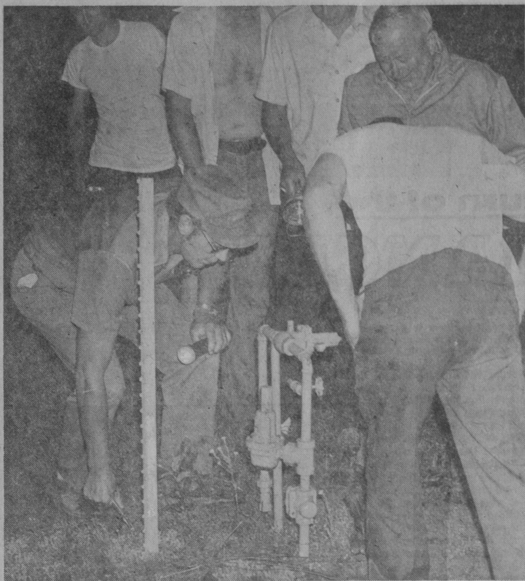
THE THEODORE ANSCHUETZ residence on M-55 had a close call during a thunder and lightning storm early last Wednesday morning. A bolt of lightning struck a regulator on a gas transmission main in front of the farm home and followed a smaller line to the house. Gas escaping from a damaged regulator scorched the side of
