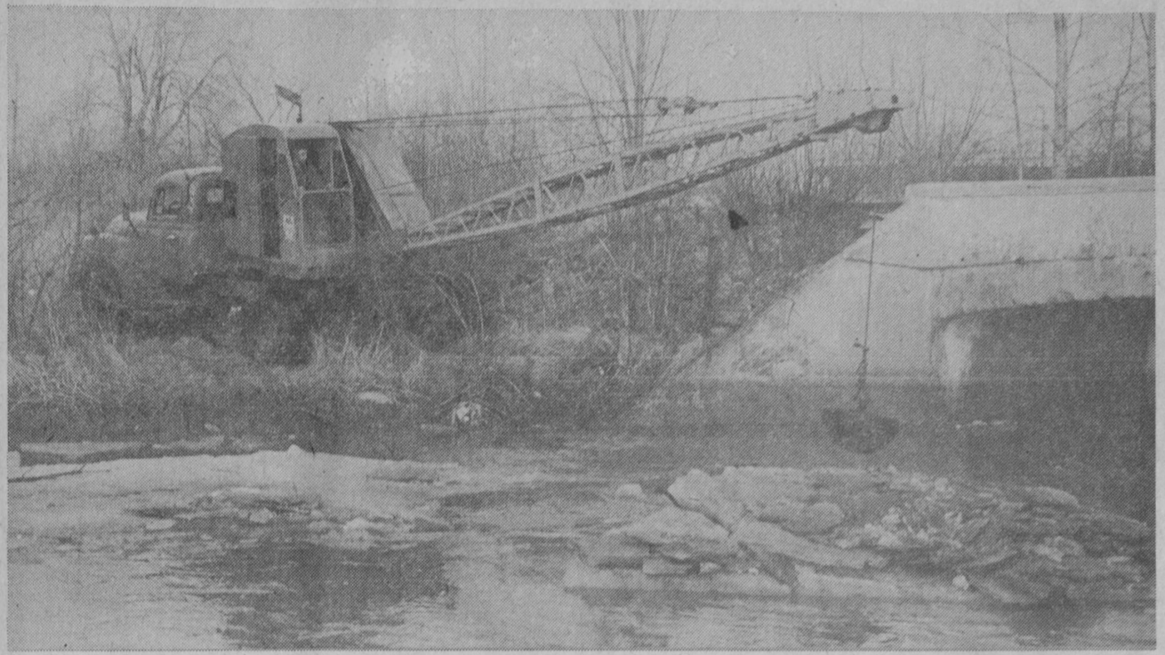
ICE BEGAN to break up last week in Dead Creek after the most severe winter in history. A dragline was used by the Tawas City Department of Public Works to prevent huge cakes of ice from jamming at the railroad bridge.—Tawas Herald Photo.
