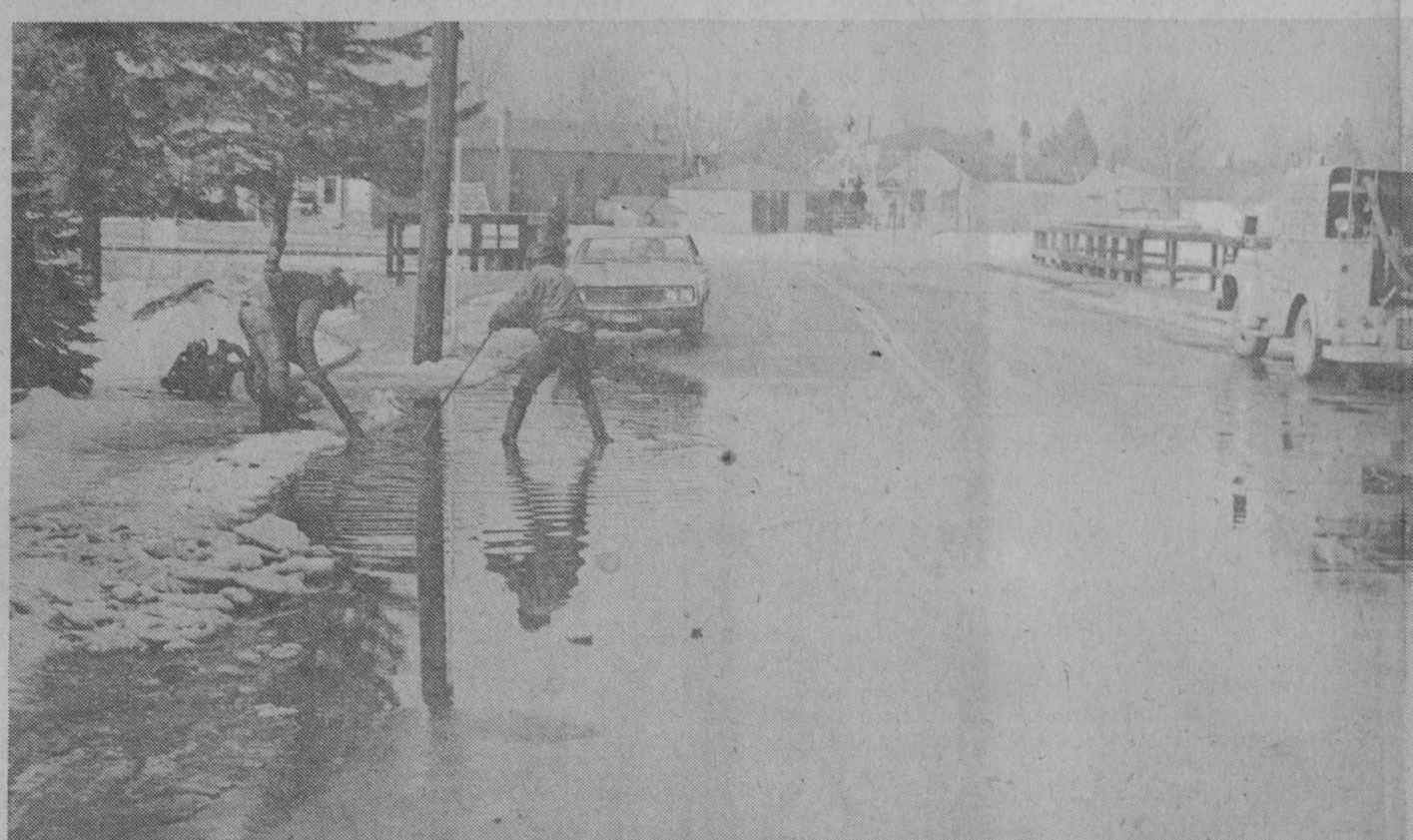
A TOUCH of what is in store for the area once spring arrives is pictured above. Two days of rain last week left large pools of water in Tawas City's Mathews Street as storm drains were frozen. Tawas City Department of Public Works utilized a portable pump in an effort to remove the water, but it was a losing battle. The worst road and street breakup in history is expected due to heavy frost penetration.—Tawas Herald Photo.
