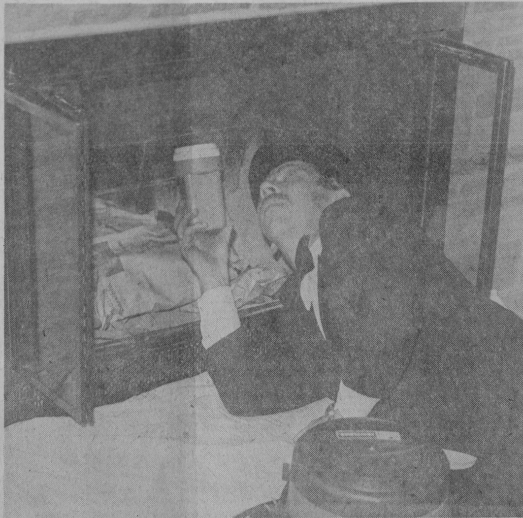
DURING CLEANING OPERATIONS, the draft of the fireplace is closed in order to prevent soot from filling the house. Hemsall is shown here as he prepares to use a vacuum to complete the work.—Tawas Herald Photo.
