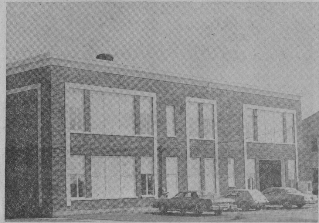
WORK is nearly completed on a $21,000 renovation at the Iosco-Arenac Regional Library headquarters at Alabaster. The project included modifying windows to conserve heat. Some of the openings were replaced with thermopane windows while other windows were completely sealed with insulated panels. A new paint job gave the headquarters building, formerly the Alabaster School, a face lifting. A fresh coat of paint was added on the interior. The project was financed through federal revenue sharing money received from the two counties. The headquarters has been located at Alabaster for the past 15 years.—Tawas Herald Photo.
