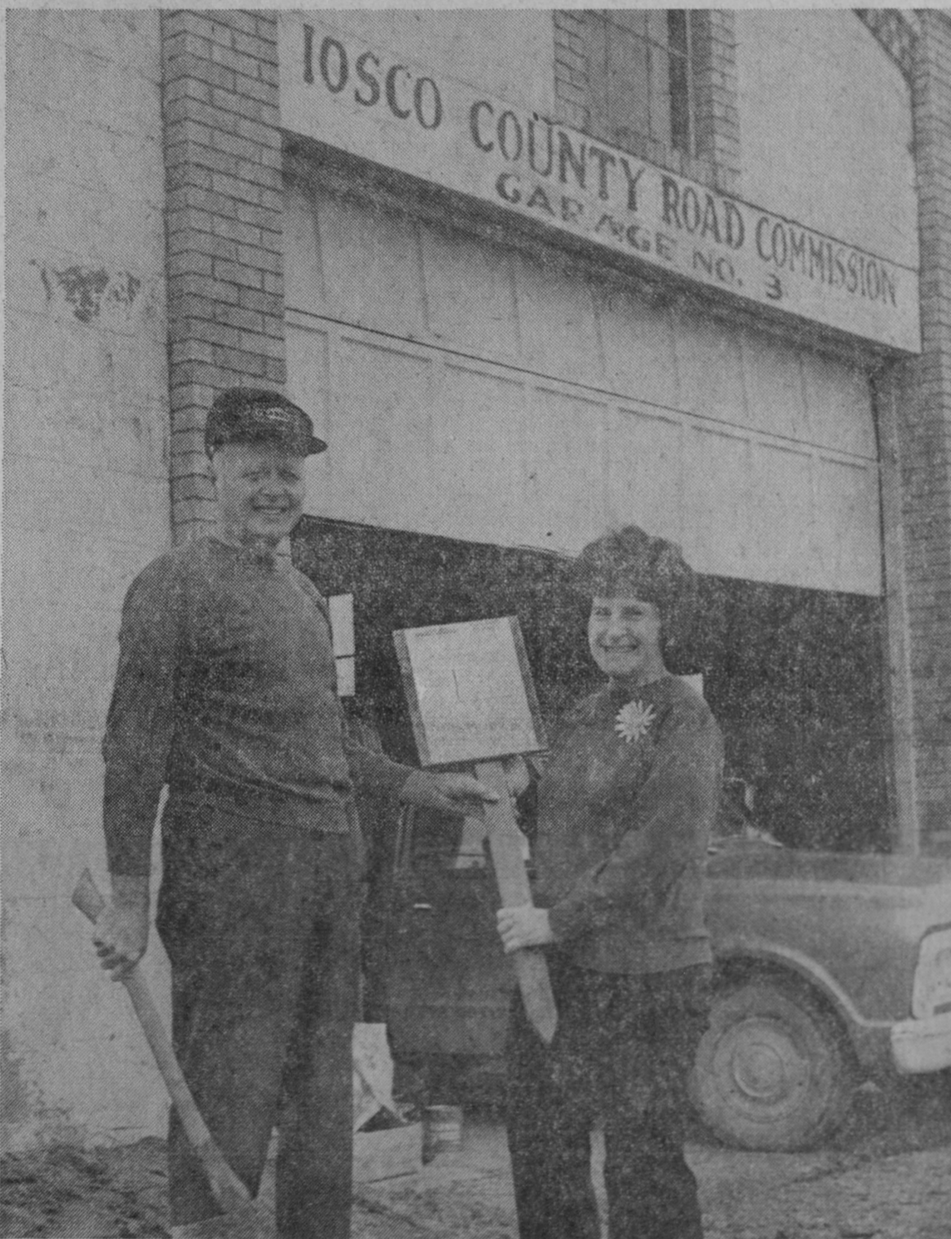
DISPLAYING the building permit for work on the new senior citizens center at Hale. The former Iosco County Garage is pictured in the background.—Tawas Herald Photo.
