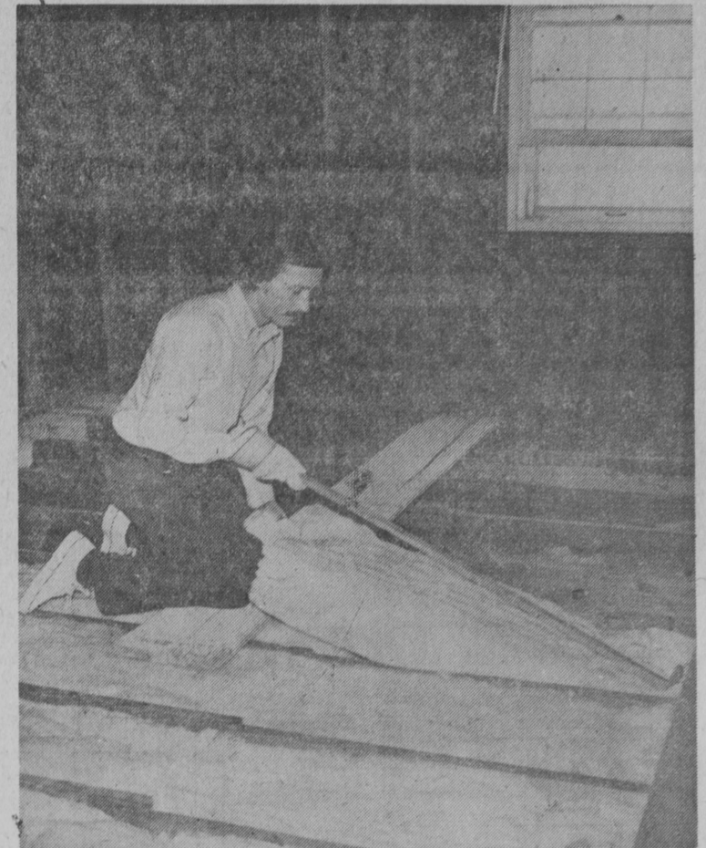
NECESSITY is the mother of invention, even when one is insulating the attic. Here is a suggestion—use a wax applicator or mop handle to help install attic insulation in hard-to-reach areas, according to the demonstration in the photograph above.
