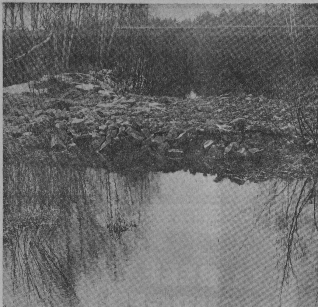
AN EARTHEN DAM was bulldozed into this canal west of Newman Street last Wednesday. The property owner, Elouise M. Dimmick, claims that the city was confiscating her property by using it for drainage.—Tawas Herald Photo.
