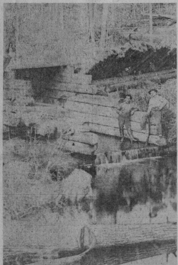
FLOODING was one means devised by lumbermen to bring their logs down the East Branch of the AuGres River. A series of sluice dams were constructed along the main stream and feeder creeks to hold back water until it reached the proper "driving pitch." Gates were opened and logs were sent down the stream. The water flow was then stopped by the gates to build up enough water for another run of logs. This was the Poscher Dam on Smith Creek in Plainfield Township. Eugene and L. B. Smith owned the water rights on this stream.
