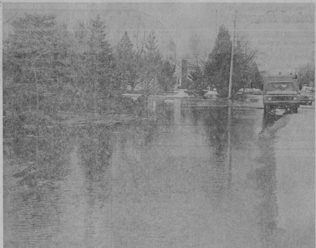
A FROZEN STORM DRAIN along First Street at the Ziel Nursery caused a large accumulation of water last week in that area. The Tawas City Department of Public Works used a portable pump to transfer the storm water across First Street and into a drain leading to Dead Creek, but thawing weather caused the drain to open Saturday night and most of the water had receded by Sunday. Two blocks east, the North Street storm drain constructed last fall had worked perfectly and there has been no flooding condition in that area this spring.—Tawas Herald Photo.
