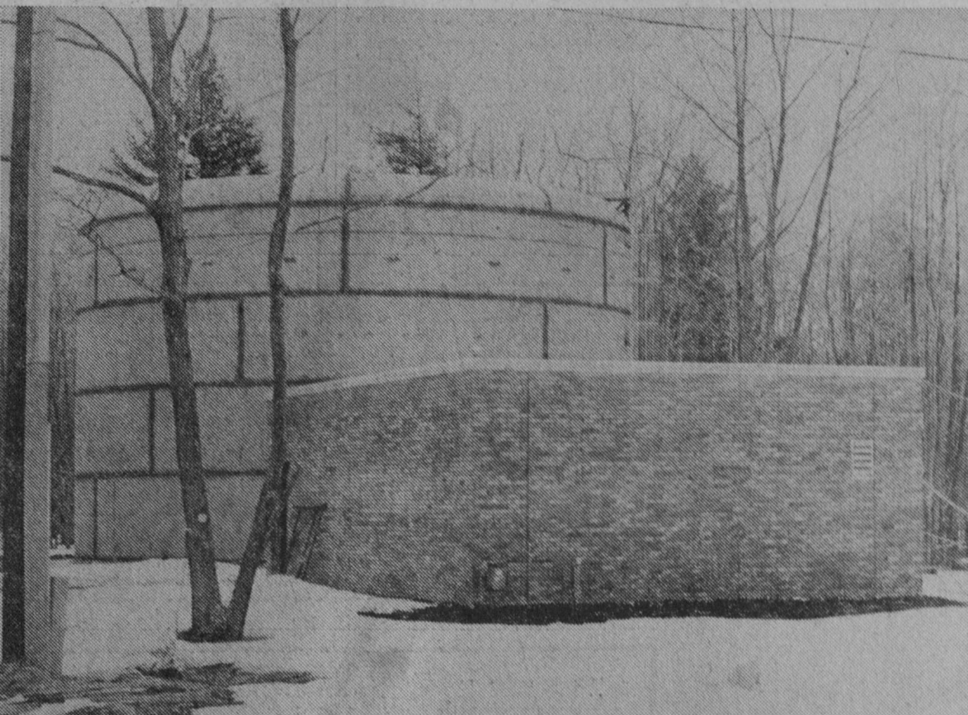
AWAITING incorporation into the expanded water system to serve the Tawas area and Baldwin Township in the spring is this new pumping station and 500,000-gallon storage tank on East Lincoln Street at East Tawas. Water from the filtration plant at the foot of Newman Street is pumped through this plant to serve the
