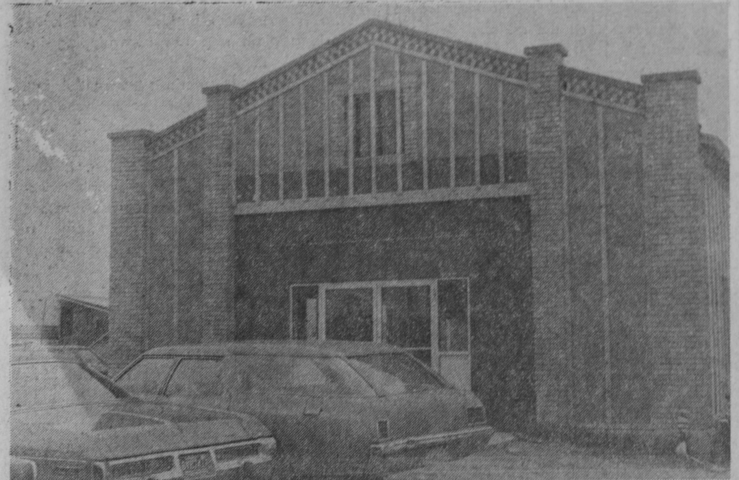
THE OLD COUNTY GARAGE at Hale awaits a covering of aluminum siding and other work
