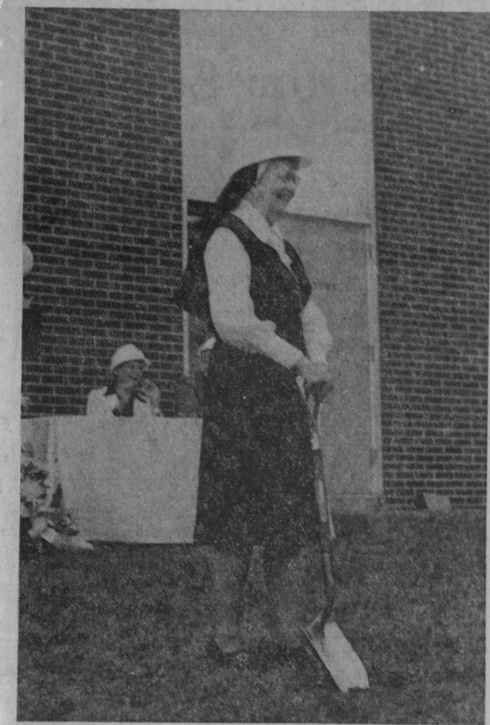
WEARING A HARD HAT for Wednesday's ground breaking ceremony at Tawas Hospital was Sister Rita Louise Sullivan, first administrator at the hospital. Turn to page 1, sec. 2, for story and pictures.—Tawas Herald Photo.
