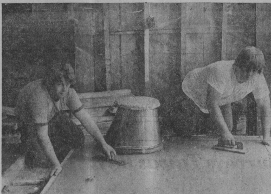
ALLEN WILSON, left, and Daniel Bergeron float cement slabs at Old Orchard Park on the AuSable River near Oscoda. Allen is in the Title III SPEDY program while Daniel participates in an inschool activity. Both are em-
