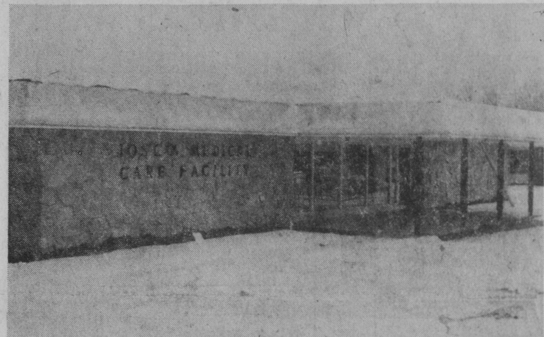
OPERATING expenses have been increasing while revenue has shown a decrease at the Isosco Medical Care Facility. Beds in the facility have a 98 percent occupancy rate. Bonds sold in 1964 to pay the county's share of the construction are being retired with the 1978 tax levy and voters may be asked to renew a portion of the millage rate to help finance operation. —Tawas Herald Photo.
