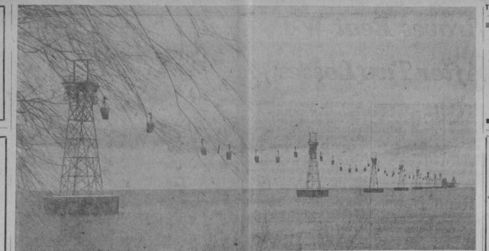
A GREAT LAKES ore carrier is shown docked at the lake crib of United States Gypsum Company's Alabaster installation as it takes on a load of gypsum ore being transferred from shore by the overhead bucket tramway system. Four more ships are to be
