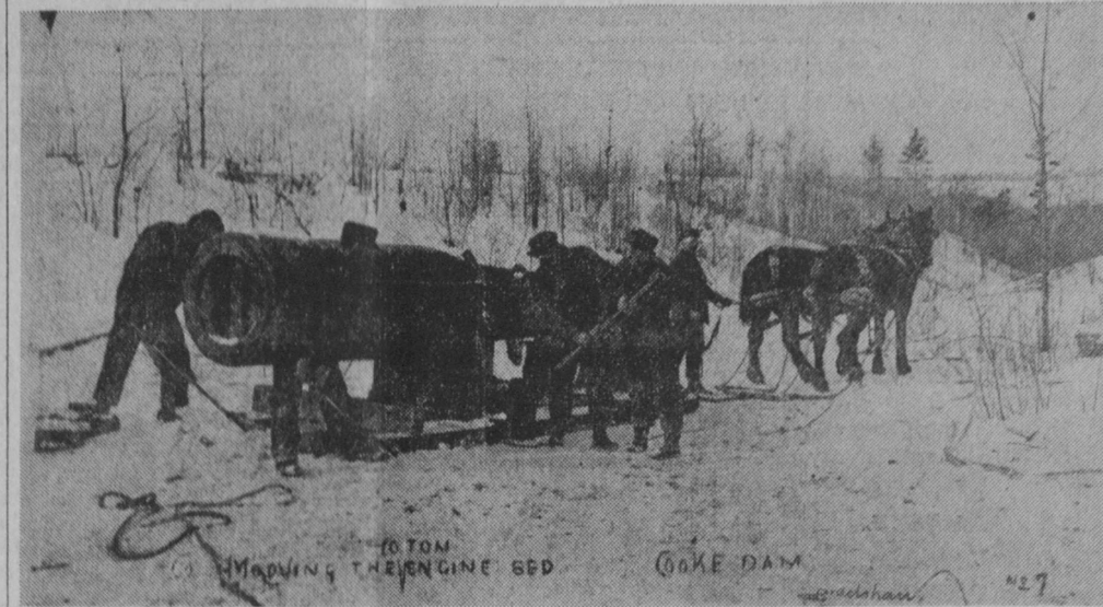
MANY HANDS and beasts were needed to move heavy equipment to the sites of dams under construction. These men are skidding a 10-ton section of a generator to the site of Cooke Dam.
