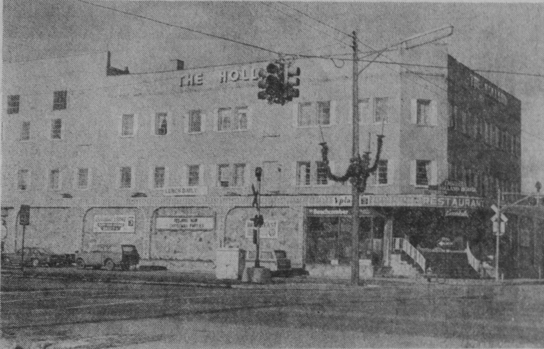
THE HOLLAND HOUSE, a landmark at the intersection of Bay and Newman Streets at East Tawas, has been declared a fire hazard by the state fire marshal and the owner has been cited
