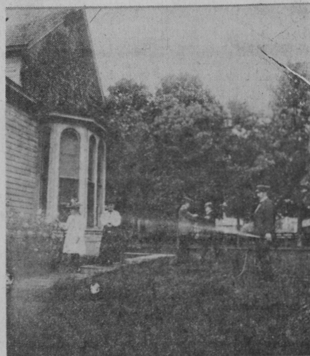
INSTALLATION of a municipal water system at East Tawas in the 1880s put an end to corner pumps and even provided an excess for watering lawns and gardens. This family was dressed in its Sunday finery when posing for A. G. Emery around the turn of the century. The father poses rather stiffly with the garden hose in one hand.
