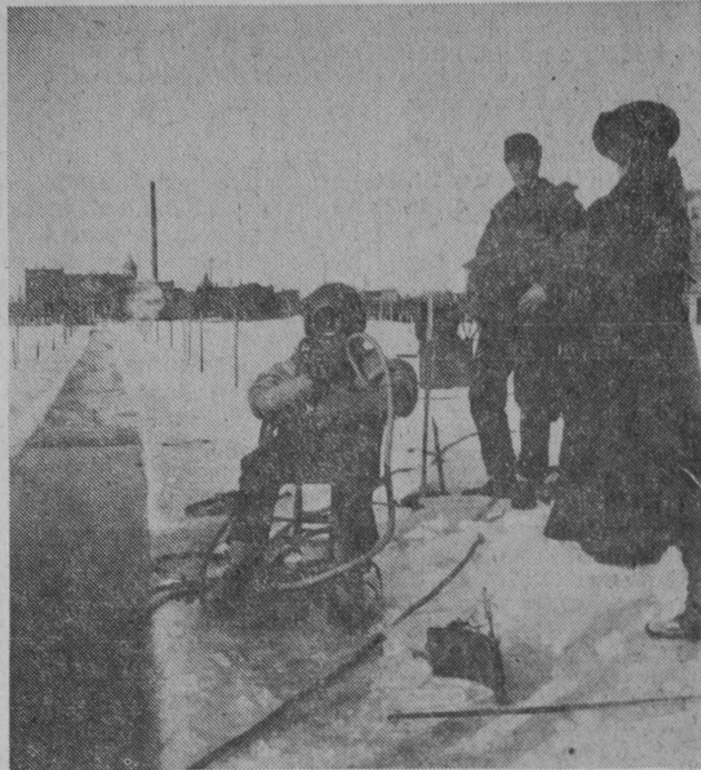
EAST TAWAS was installing a new water intake when this picture was snapped. Buildings in the picture date it around 1904. The smokestack to the right of the Holland Hotel served the municipal generating plant which provided electricity to the community. The hardhat diver is preparing to inspect the cast iron pipe, which had been assembled on the ice and then lowered to the lake bottom.
