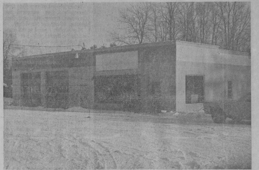
FRONT of the new branch library in Tawas City is pictured above. The building formerly served as a recreational vehicle sales, a garage and a restaurant.—Tawas Herald Photo.
