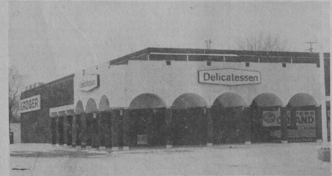
DISTINCTIVE entrance arches of the new Kroger Superstore in Tawas City are shown above. Formal grand opening of the store is to start Sunday with a ribbon cutting ceremony at 9:00 a.m.—Tawas Herald Photo.
