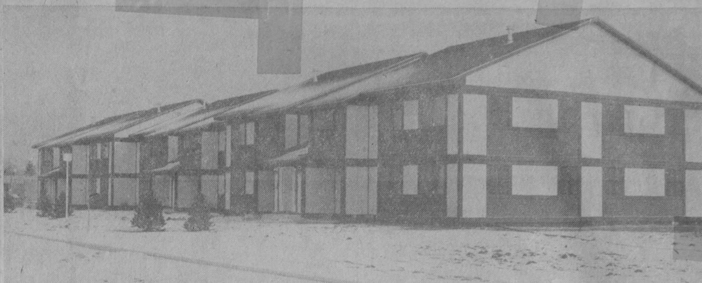
Manitou Village apartment complex under construction.
