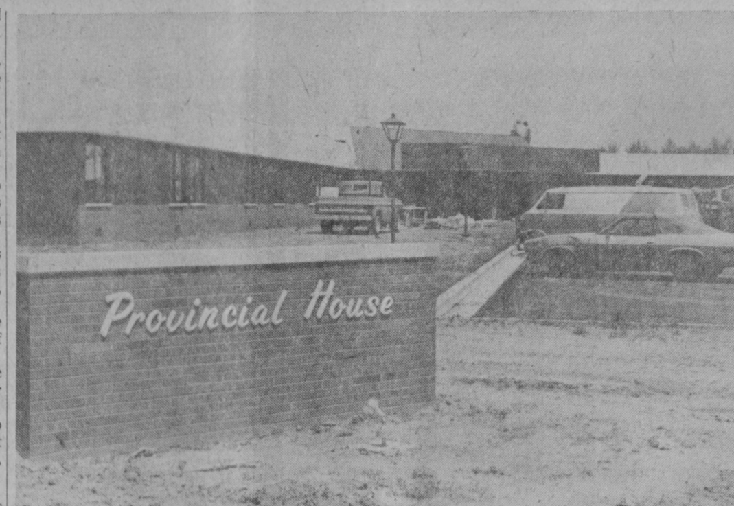
WORKMEN were installing metal on the front of the new Provincial House skilled nursing home last week as preparations were being made for an open house. Construction of the facility was started last fall.—Tawas Herald Photo.
