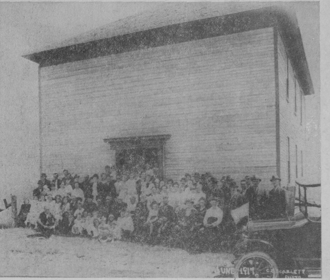
ORANGE HALL across from the Hemlock Road Baptist Church served a dual purpose in the early 1900s. The second floor was used as the meeting place for the Grant Heroes No. 456, Orange Society, and the ground floor was for public meetings and community dances. The above group picture snapped by C. E. Scarlett in 1917 shows members of the Isosco County Pioneer Society during that group's annual meeting.—Tawas Herald Photo.
