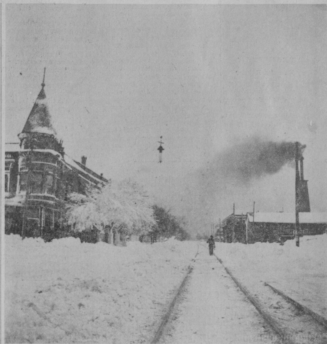
TWO WORKMEN were killed and two were injured when a steam boiler exploded in one of the buildings at right at East Tawas on November 18, 1912. Bodies of two of the men were hurled across Bay Street; a third man was
