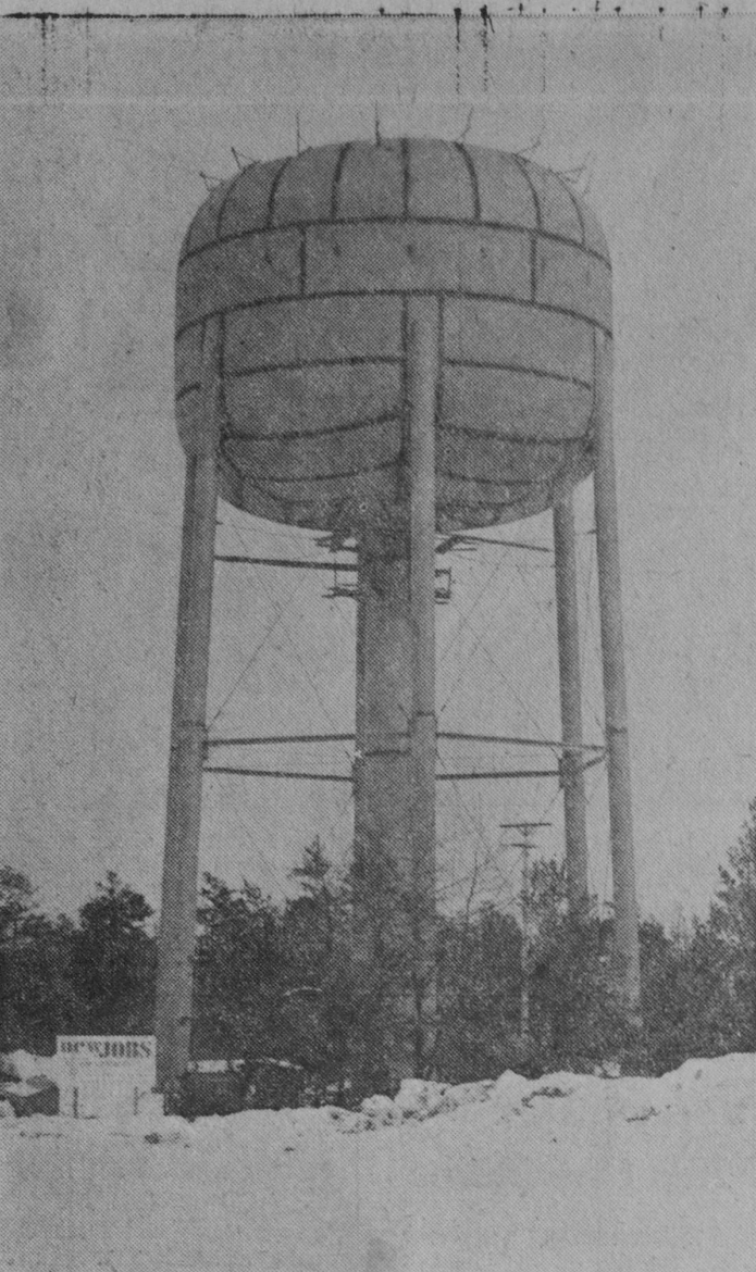
A WORKMAN fell 150 feet to his death Thursday afternoon during the final phase of construction on this water tank at the Tawas Area Industrial Park in Baldwin Township. A similar water tank was constructed at the Tawas City industrial park without incident.—Tawas Herald Photo.
