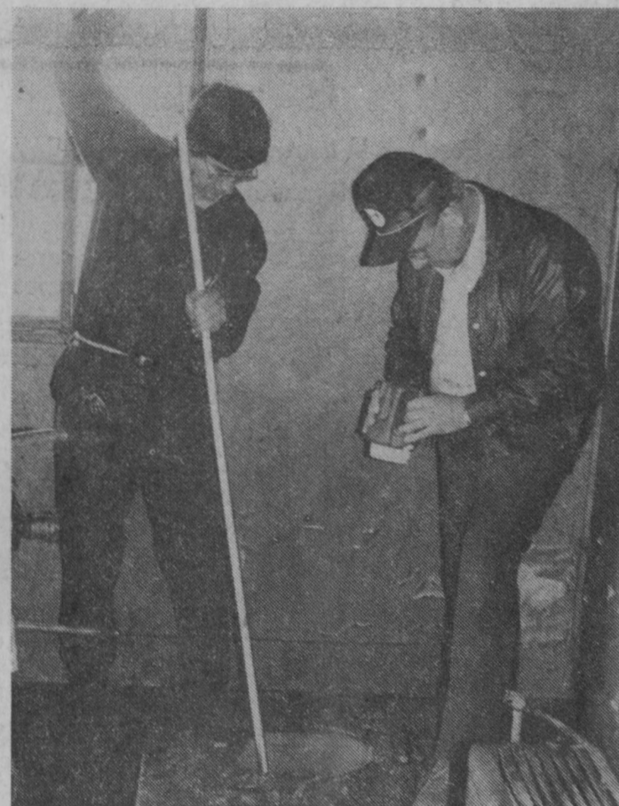
CHECKING the buildup of scale on walls of the 10-inch well casing are Theodore (Ted) St. James and Reginald Bublitz. It was hoped yesterday (Tuesday) that a submersible pump nine and three-quarters inches in diameter could be lowered inside the well.—Tawas Herald Photo.
