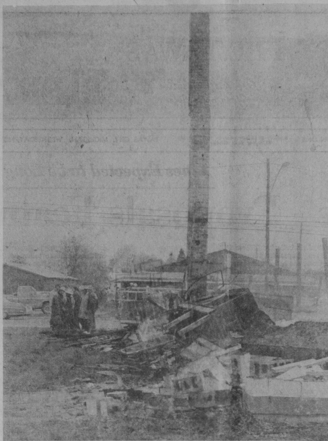
A CHIMNEY sticks out of the rubble of an unoccupied commercial building at Whittemore after last Wednesday morning's fire. Firemen at left are awaiting the arrival of the state fire marshal to begin investigation of suspected arson.—Tawas Herald Photo.
