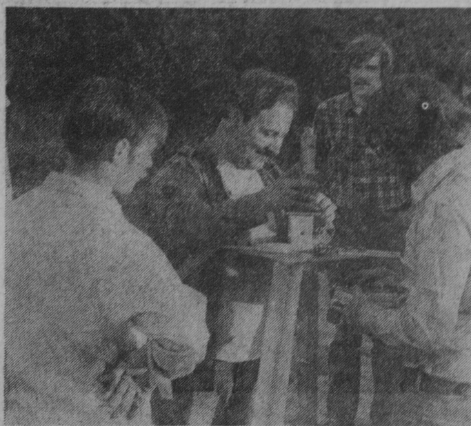
THESE WORKMEN are preparing an installation for new space age technology in the Tawas area. Turn to page 5 for another picture showing what they are doing.—Tawas Herald Photo.
