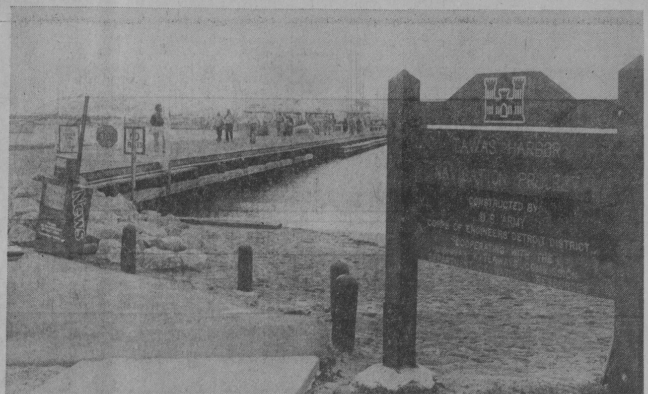
MICHIGAN WATERWAYS COMMISSION DOCK at East Tawas has been a busy place during the past summer with large numbers of fishermen enjoying the new pier facilities in Tawas Bay. The harbor master's office reports that the Labor Day week-end saw the most active use of the season by small craft. It is expected that the fall fishing season will continue to see extensive use of the new facilities, despite the fact that the state has not improved parking facilities at the installation.—Tawas Herald Photo.
