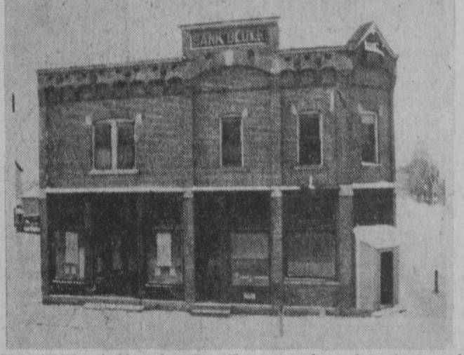
THE FIRST switchboard at East Tawas was located on the second floor of the old Bank Block, now a meeting room over the law office of Michael Freel and Thomas Huck.
