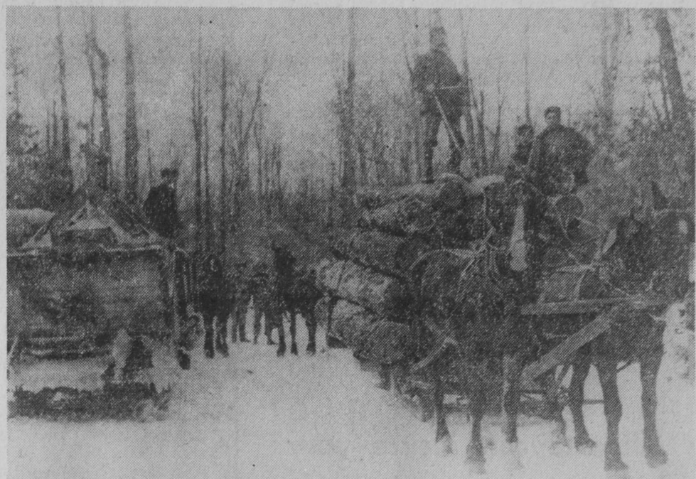
HEADING for a banking ground in Plainfield Township, this team and sledge load of logs skims over an ice road, especially prepared for logging purposes. A sprinkler sledge is at left. The wooden tank was filled
