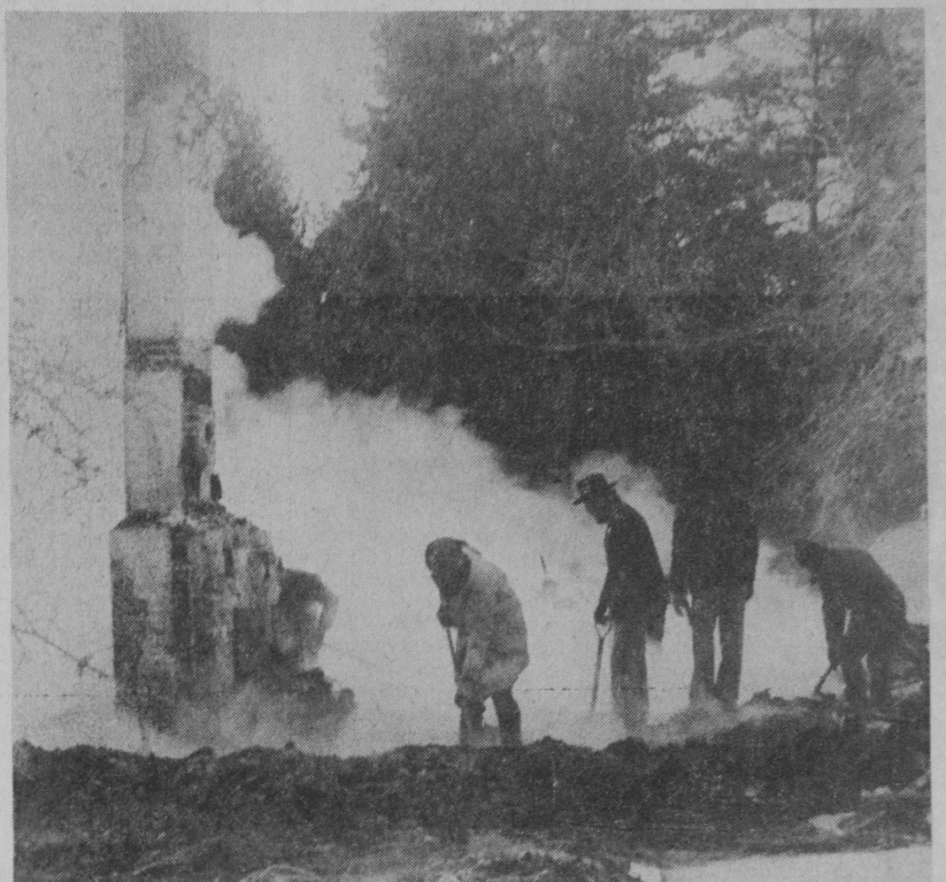
FIREMEN and sheriff's department deputies were sifting through debris in search for the body of a home fire victim early last Thursday morning in Alabaster Township. Only the fireplace chimney was standing after the blaze.—Tawas Herald Photo.
