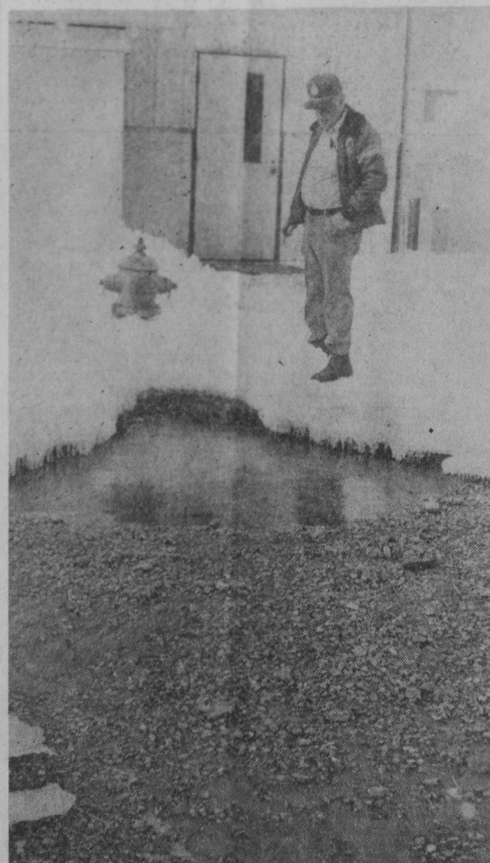
SURVEYING the damage caused early Sunday when vandals opened a fire hydrant behind Tawas Area High School is Merlin Look, superintendent of public works of Tawas City. A fire hydrant was also opened Sunday at East Tawas causing a flooded condition on Lincoln Street.—Tawas Herald Photo.
