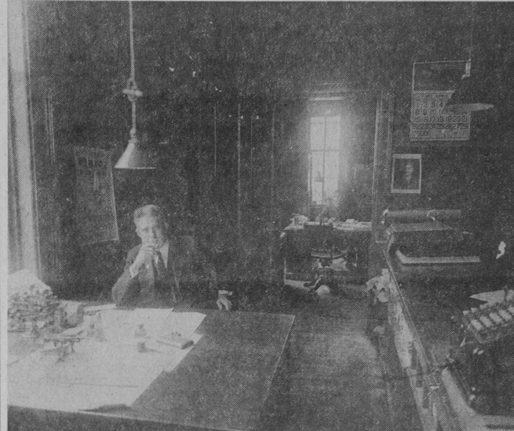
THIS IS THE ONLY KNOWN view of the interior of the old Iosco County Courthouse in Tawas City. It shows Joseph G. Dimmick seated at his desk in the county treasurer's office. Through
