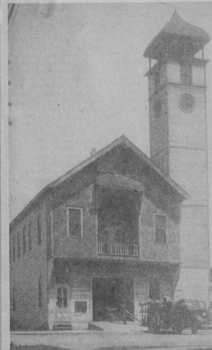
THE UNIQUE ARCHITECTURE of the old East Tawas City Hall is shown here. If it was standing today, it would be listed on both state and national historic building registers. The tower was used by the fire department to dry hoses.
