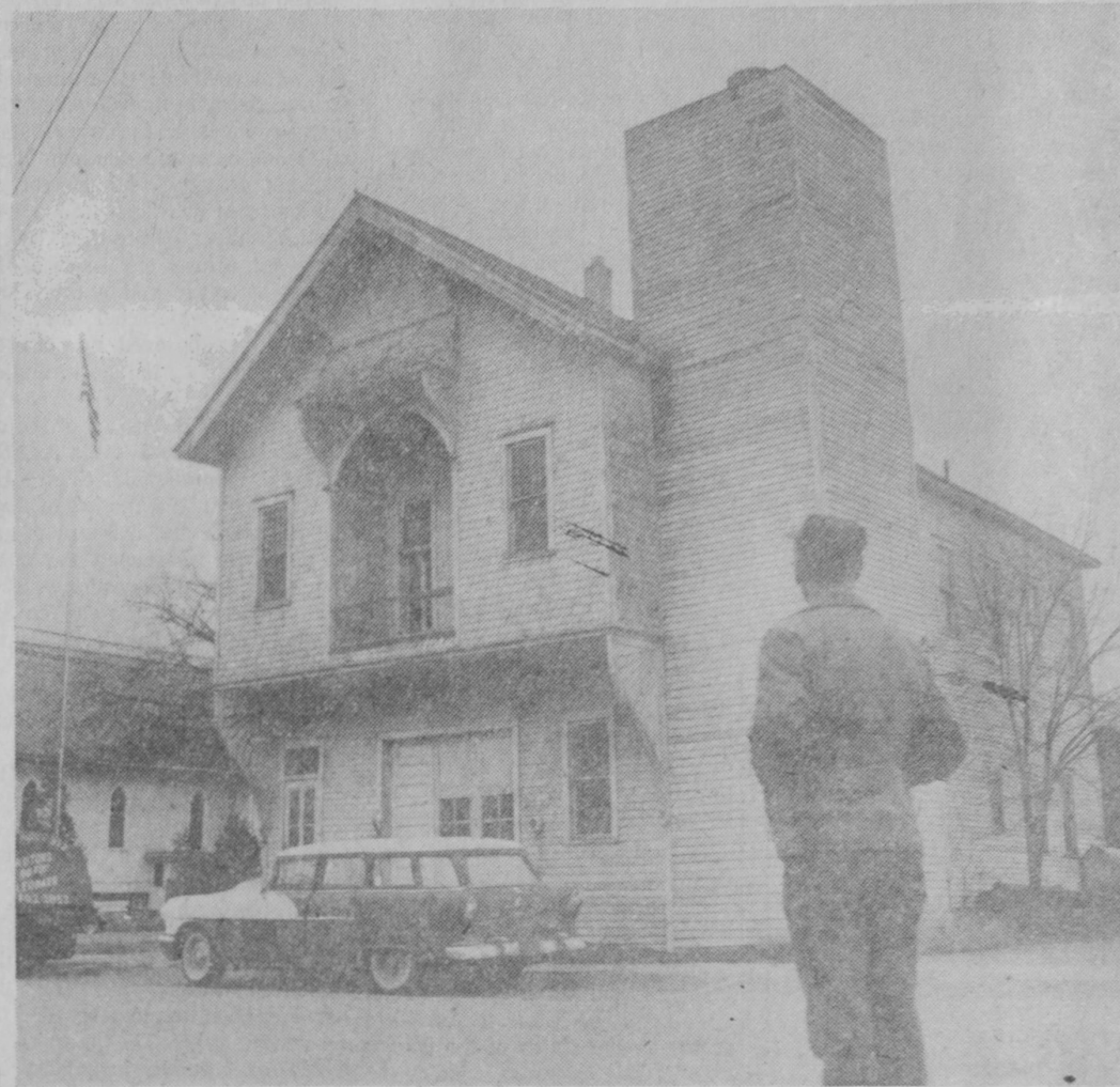
REPLACEMENT of the old East Tawas City Hall provided that community with several years of controversy from 1959 to 1962. Paul Koper, who was city superintendent at the time, is surveying the old building prior to the start of demolition in 1961.—Tawas Herald Photo.
