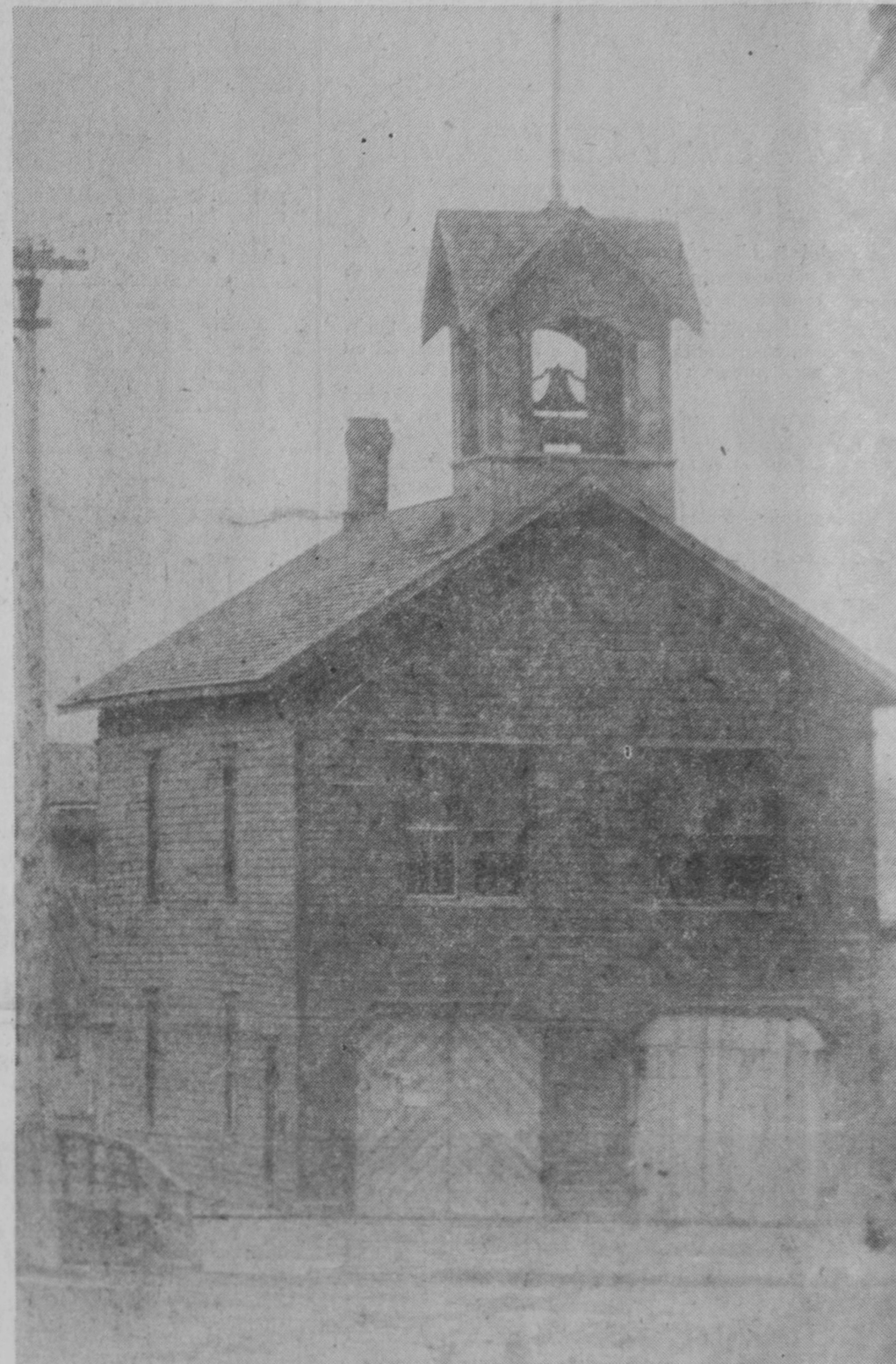
THIS TWO-STORY frame building, located at the northeast corner of the Mathews Street bridge, served as the seat of municipal government in Tawas City until 1925. The bell in the tower served as the city's fire alarm and fire apparatus—first a hand pumper and a hose cart—
