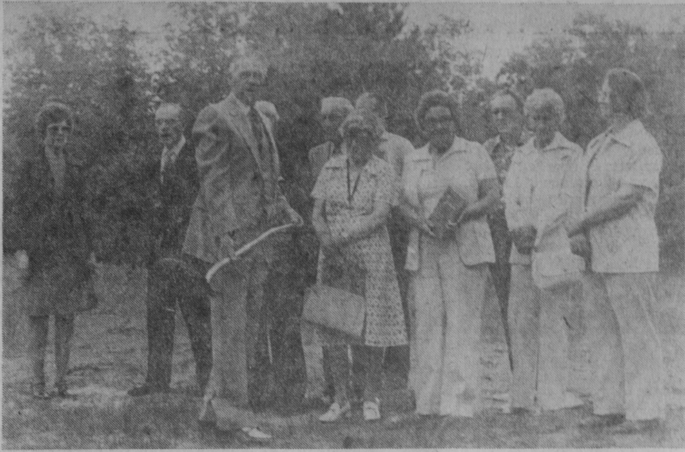
GROUND was broken Sunday morning for the Wilber United Methodist Church. Shown with the shovel is the Rev. Clifford DeVore, with church trustees and members of the building committee watching.—Tawas Herald Photo.
