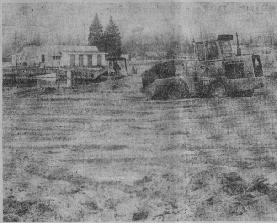
AFTER MONTHS of discussion and waiting for a permit from the federal government, work was finally started last Friday on filling the old boat slip at the mouth of the Tawas River. The original boat slip was excavated in August 1934 by the late Joseph Lubaway when the property was owned by the Tawas Yacht Club. The property was purchased by the city less than two years ago and sand which had been removed in past river dredging operations was pushed into the slip. The city awaits word on federal and state grants for development of the property for recreational use.—Tawas Herald Photo.
