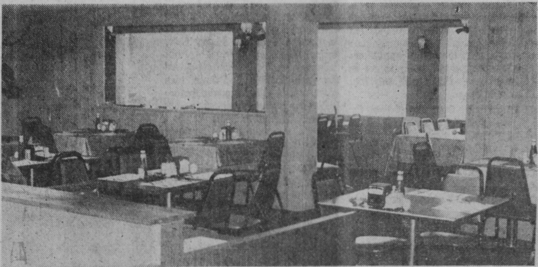
GRAND OPENING of the newly remodeled and expanded Coyle's Restaurant in Tawas City is to be held April 1, 2 and 3. The dining room area was expanded, new picture windows were installed overlooking Tawas Bay, along with new carpeting, new rest-rooms and booths.—Tawas Herald Photo.
