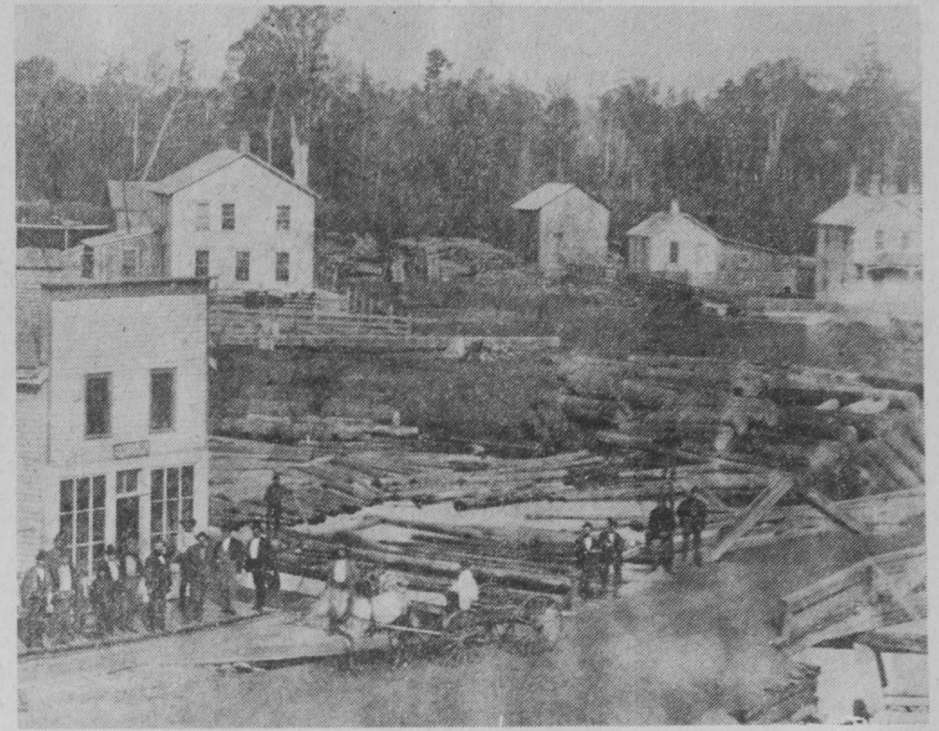
THE MEN AT RIGHT are standing on the approach to the Mathews Street bridge over the Tawas River. The original picture was copied into postcard size about 70 years ago and surviving prints list both 1868 and 1873 as the date of the original exposure. A temporary bridge preceded this structure. The Tawas River below the bridge is jammed with pine logs bound for the Whittemore mill. Men at left are standing in front of a saloon.—Copy by August Brown.
